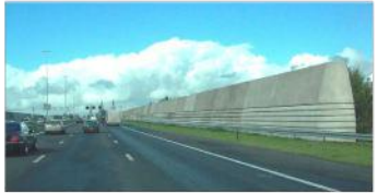
Dutch concrete noise barrier bent at a small angle from the road in order to reflect the noise upwards to reduce the disturbance of residents on the other side of the highway. Source: "Noise Barrier Design" Hans Bendtsen
