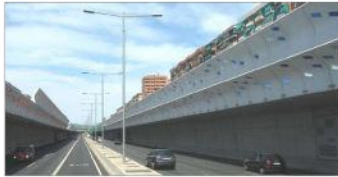
Precast concrete noise barriers with colored transparent openings bending over the highway in Barcelona. The shape of the geometry limits noise diffraction on to the buildings. Source: "Noise Barrier Design" Hans Bendtsen
