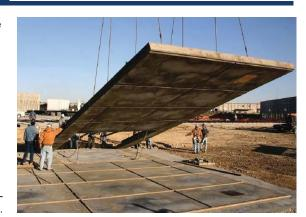
Panel is horizontally casted with wood formwork on floor slab
